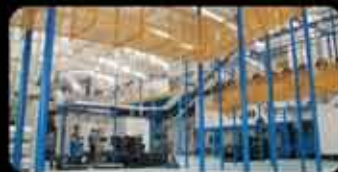
Automated Painting system. Capacity 100,000 pieces
